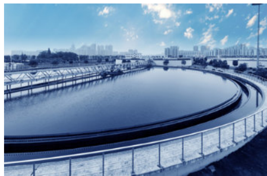
Effluent Treatment Plant
